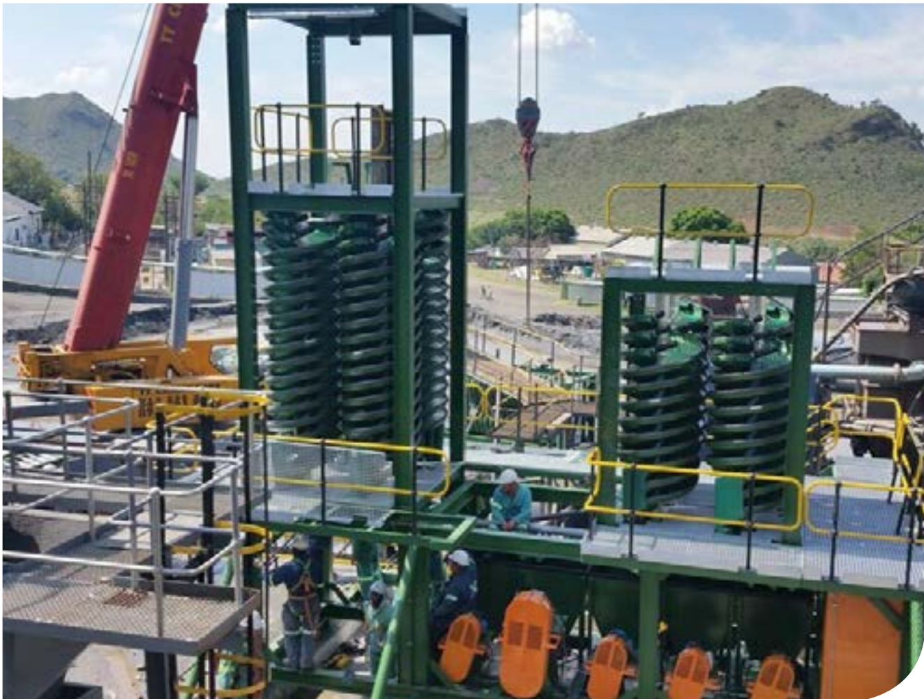
Dilokong Chrome beneficiation under construction
