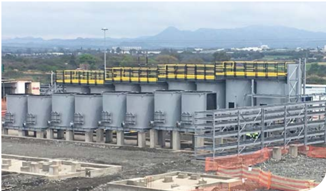
Hernic Tailings Project – beneficiation plant
